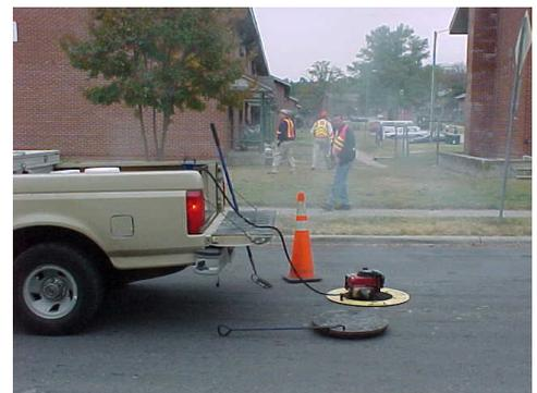
Smoke testing the collection system during a PIT Stop
