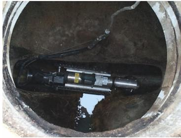
A sewer camera in a manhole during a PIT Stop
